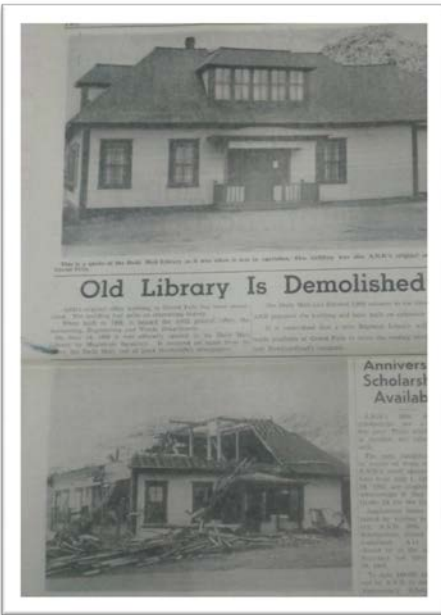
The original general office was demolished in the Spring of 1962
