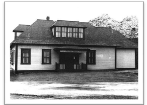
The original general office of the Anglo-Newfoundland Development Company
